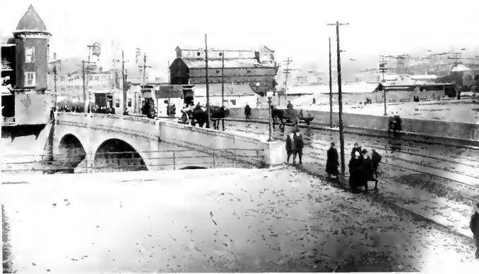
THE BROOKLYN BRIDGE, CARRYING BANK STREET OVER THE NAUGATUCK RIVER
